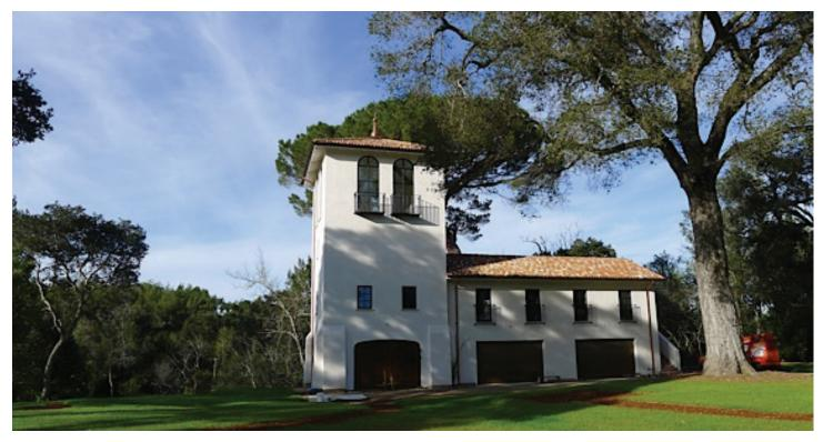
This Woodside Retreat includes a demolition of a historic main house and retention and re-purpose of the water tower and existing spaces above the garage. PARADIGM was selected to provide structural design for the existing water tower. This included a new wood framed structure replicating the original water tower structure. This new structure consists of "stacked" walls and floor framing such that usable space would be provided for the caretaker's residence.
