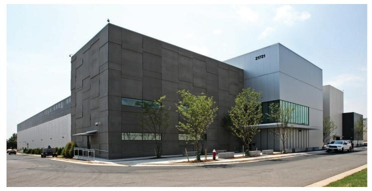
PARADIGM was selected to assist the Engineer of Record on behalf of the Owner for this 18 MW, 110,000 gsf two-story, tilt-up concrete slab on grade LEED certified building. This structure houses offices, customer support areas, colocation space, and electrical and mechanical equipment rooms. PARADIGM designed the foundation for this building which incorporated straight shaft piers ranging in depths from 4' to 25'.
